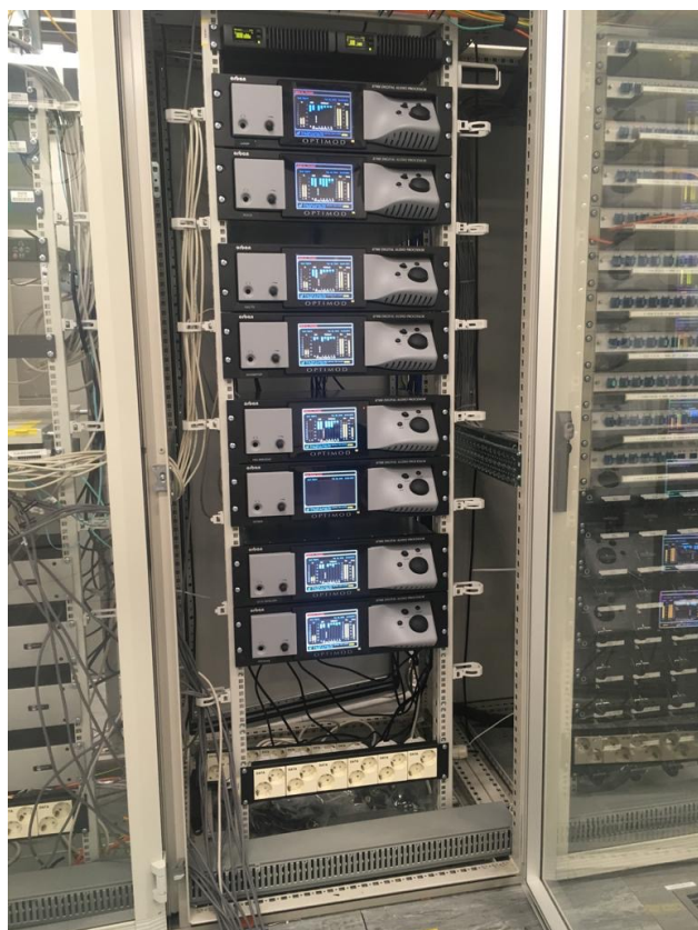
Rack with OPTIMOD 8700i Audio Processors
